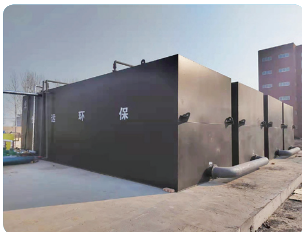
Shandong Heze School Sewage Treatment Project
