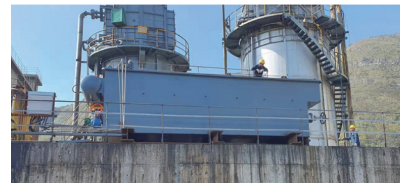
Chenzhou, Hunan - Chemical Plant Sewage Treatment Project
