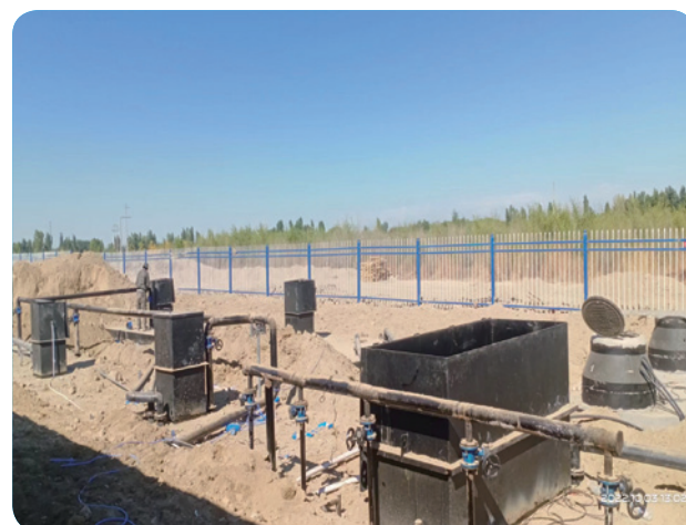
Xinjiang Yili Hospital Sewage Treatment Project
