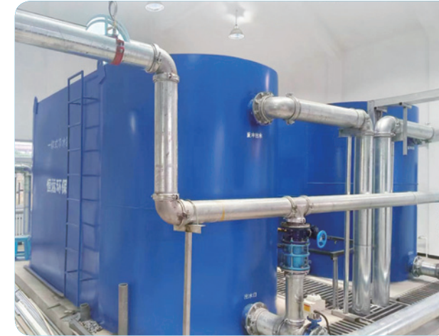
Liaoning Fushun 720-ton water plant project
