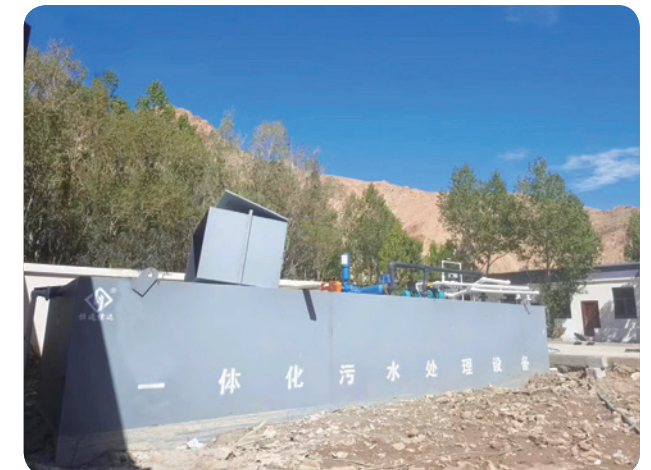
Tibet Mountaineering Training Camp Domestic Sewage Treatment Project
