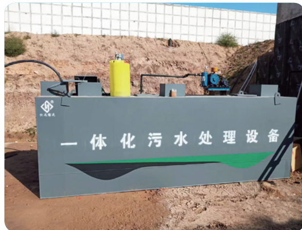
Inner Mongolia Chifeng Enterprise Sewage Treatment Project
