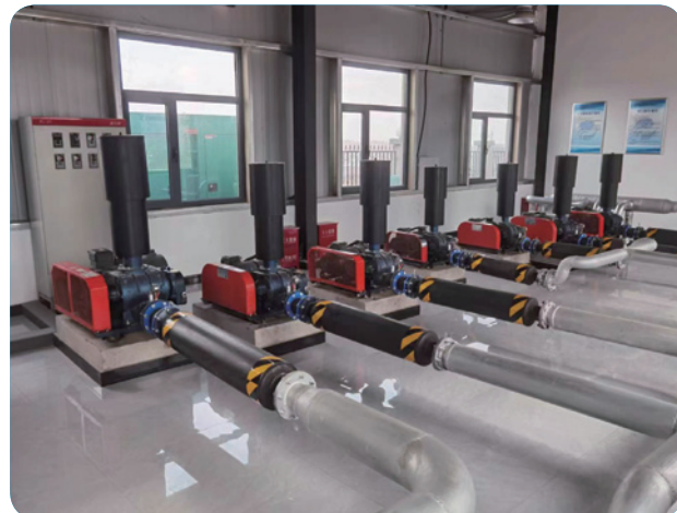
Wastewater Treatment Plant Project in Lanzhou New Immigrant Area
