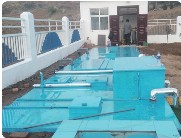
Shanxi Jincheng Wastewater Treatment Plant Project
