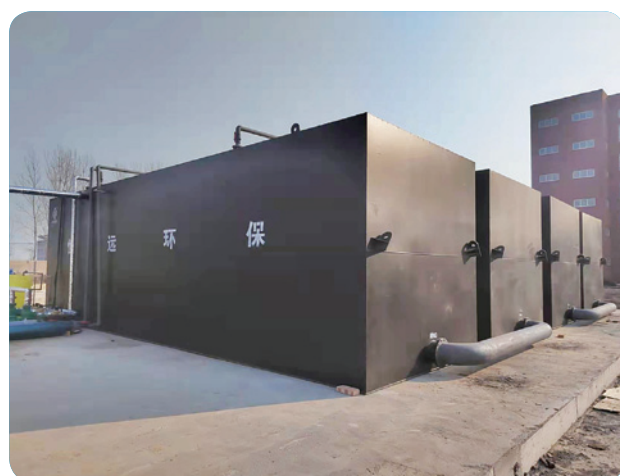
Shandong Heze School Sewage Treatment Project
