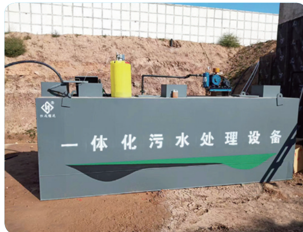
Inner Mongolia Chifeng Enterprise Sewage Treatment Project
