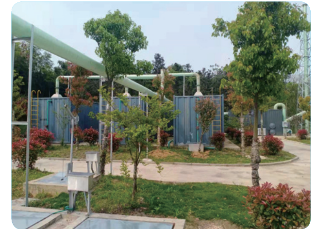
Anhui Langxi 500 mt/d domestic wastewater treatment project
