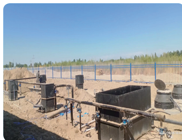
Xinjiang Yili Hospital Sewage Treatment Project
