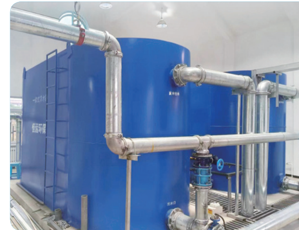
Liaoning Fushun 720-ton water plant project
