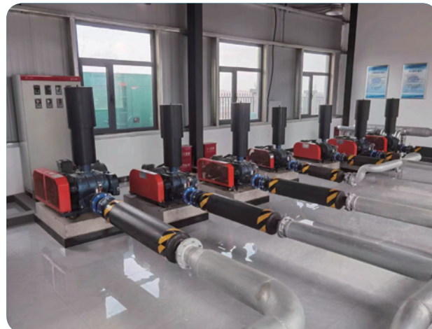
Wastewater Treatment Plant Project in Lanzhou New Immigrant Area
