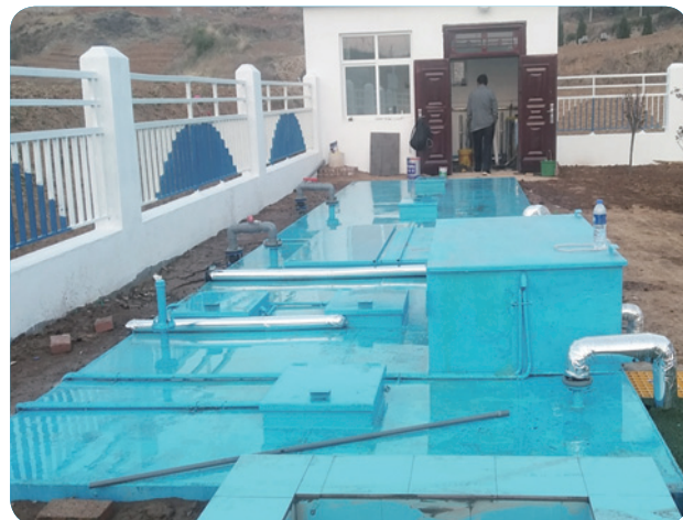
Shanxi Jincheng Wastewater Treatment Plant Project
