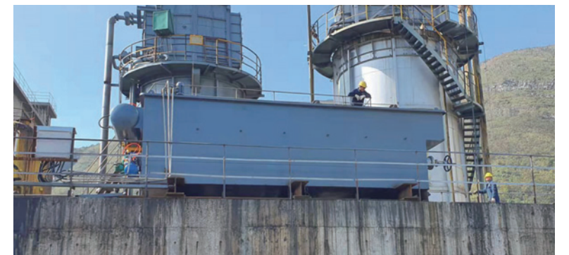
Chenzhou, Hunan - Chemical Plant Sewage Treatment Project
